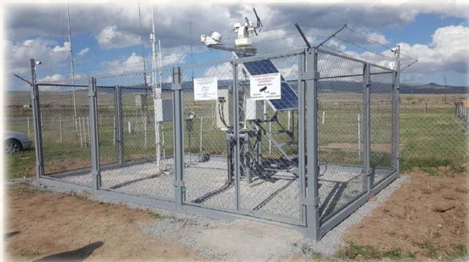
Typical field installation of SEMS-3000 System with solar sensors mounted on the sun tracker, plus meteorological mast, data-logger and power supply for autonomous unattended operation of the whole system
